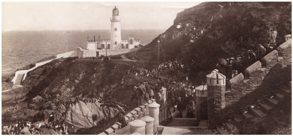
Douglas Head Lighthouse [photo by kind permission of Manx National Heritage]
