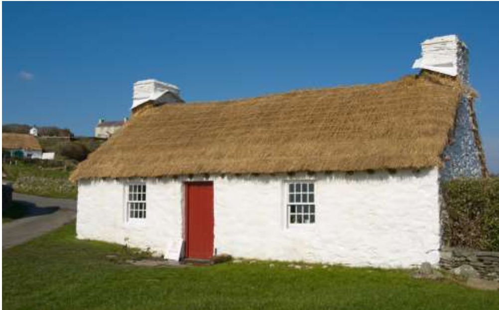
Harry Kelly's Cottage in Cregneash Village
