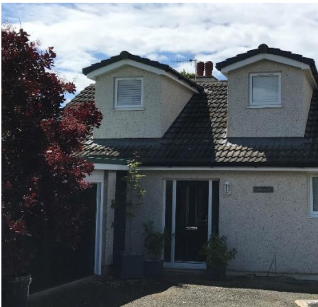
Front access from Driveway
