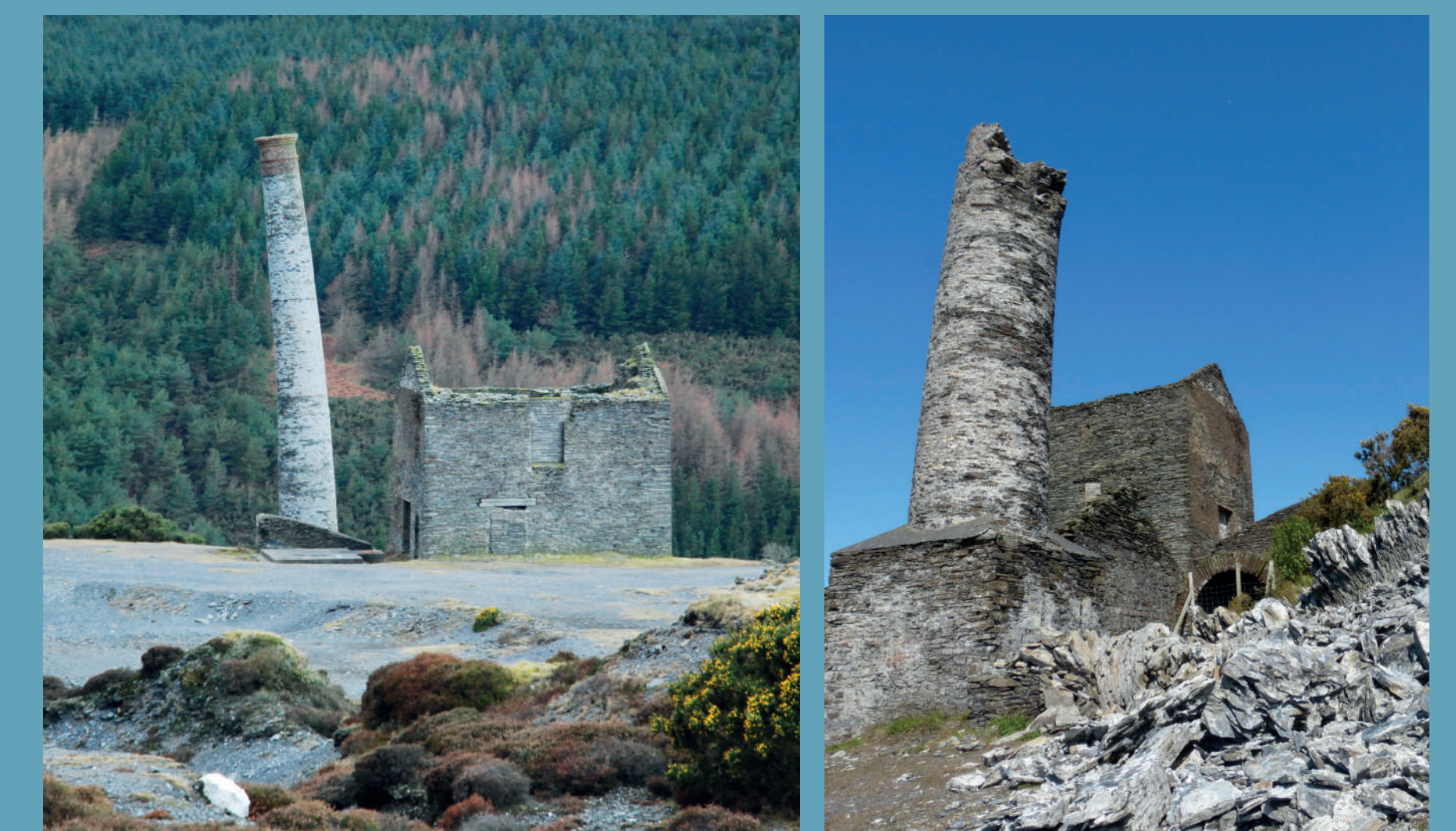
Fig.2—Beckwith's leaning chimney before collapse (left); after collapse (right). Images courtesy of Manx Scenes (left) and Energy FM (right)
